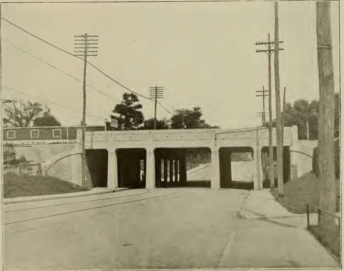
E. Washington Street, Indianapolis, Indiana. Improper treatment of a main thoroughfare.
